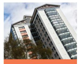
"These blocks, constructed during the early 1960s, had no wall insulation while the windows were single glazed and in poor condition. By carrying out the substantial improvements it is estimated that, in total, approximately 9600 tonnes of carbon dioxide emissions will be saved every year."
