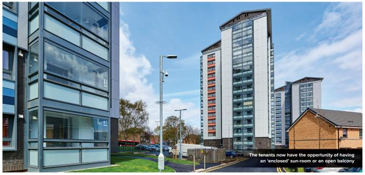
the homes had no wall insulation and were single glazed. As a result of the refurbishment, an insulated cladding system has been installed together with new energy-efficient windows and the former concrete balconies have been transformed into stunning balcony enclosures. These new balconies, manufactured by Windoor UK, have totally transformed the external façade, which also contributes to improving the visual appearance of the wider area.
